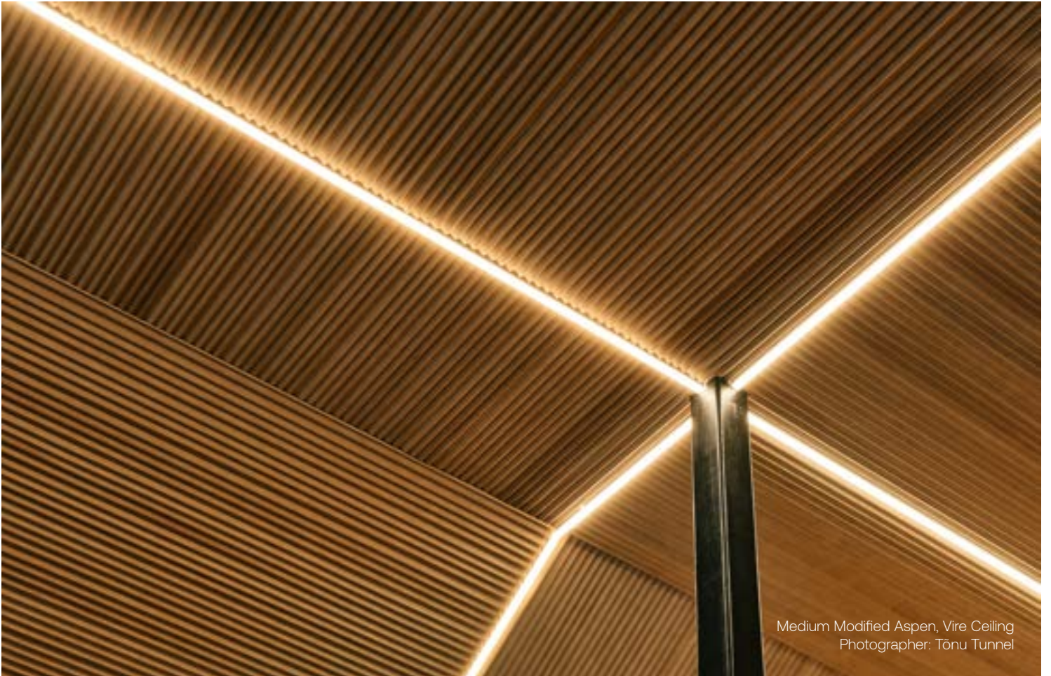
Medium Modified Aspen, Vire Ceiling, Clear Pine Dividers Photographer: Tõnu Tunnel
