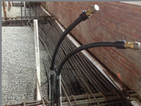
The flexibility and long lengths of TracPipe PS-II allowed for a total install time of just 36 hours versus an estimated 1200 hours for black iron pipe.
