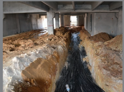
Through parking garage for new apartment complex.
