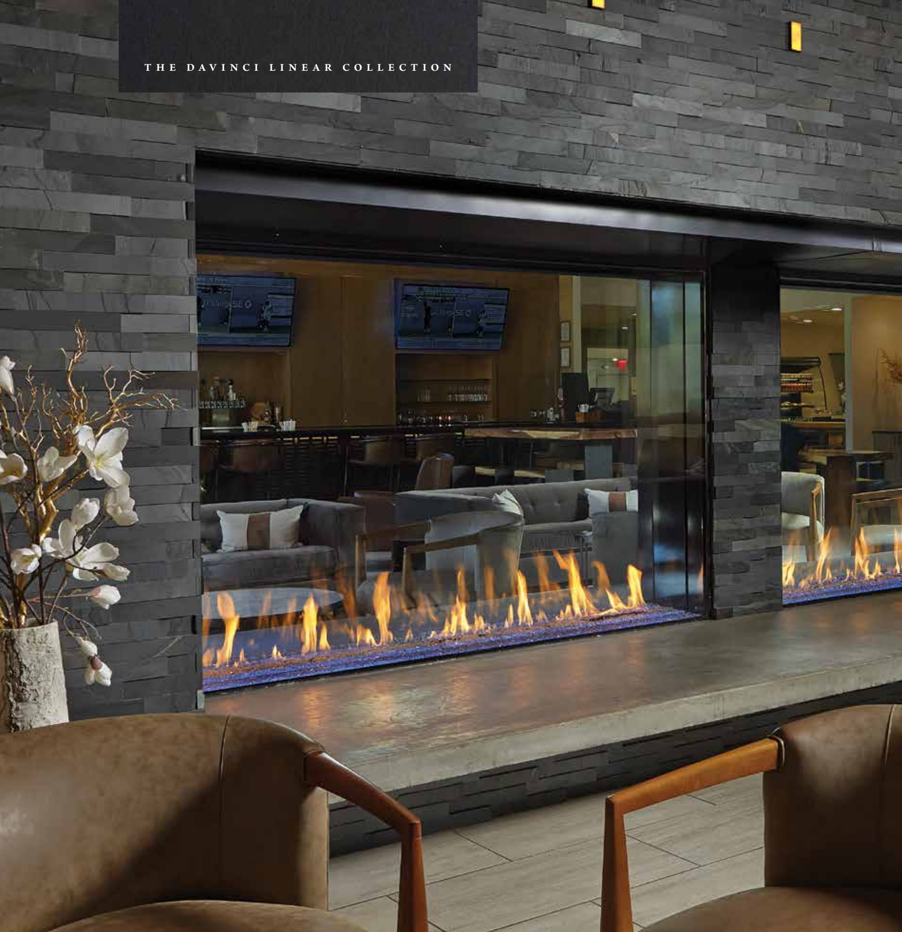
TWIN 96 X 58 INCH SEE-THRU FIREPLACES CREATE A DRAMATIC SPACE SEPARATION IN THIS HILTON DOUBLETREE, LOCATED IN VAIL, CO.
