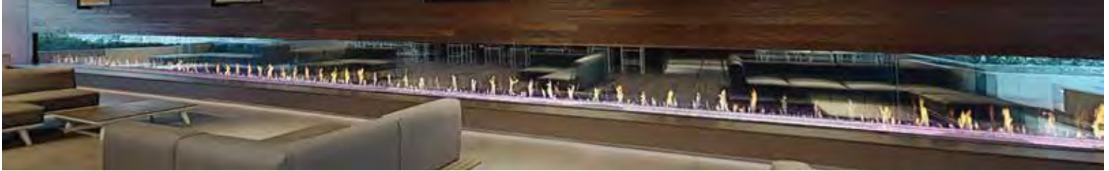
66-FOOT SINGLE-SIDED DAVINCI INSTALLED AT THE DEAN APARTMENTS, MOUNTAIN VIEW, CA
